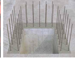
Post Installed Rebar Connections
